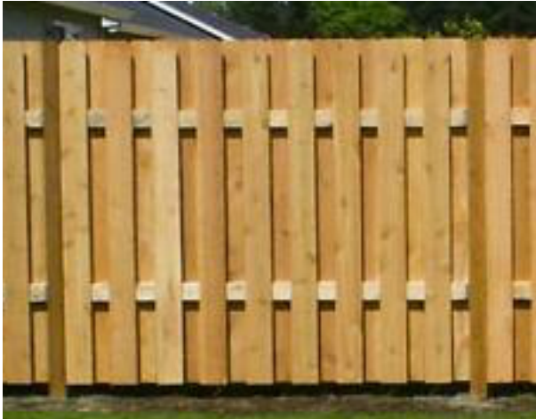
Shadow-Box Privacy (Wood or Composite) May only be used in certain cases
